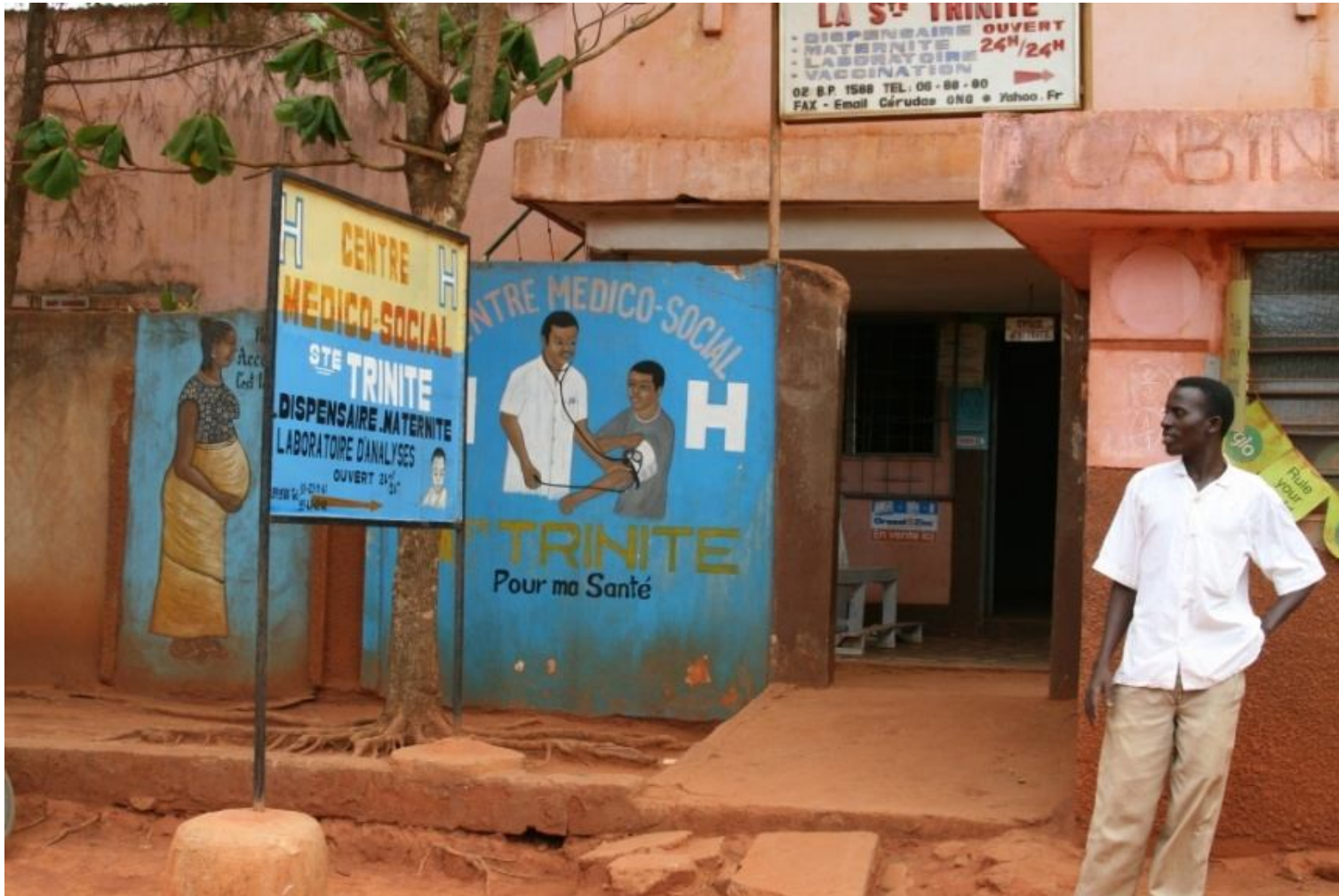
NGO Health Facility, field practice
